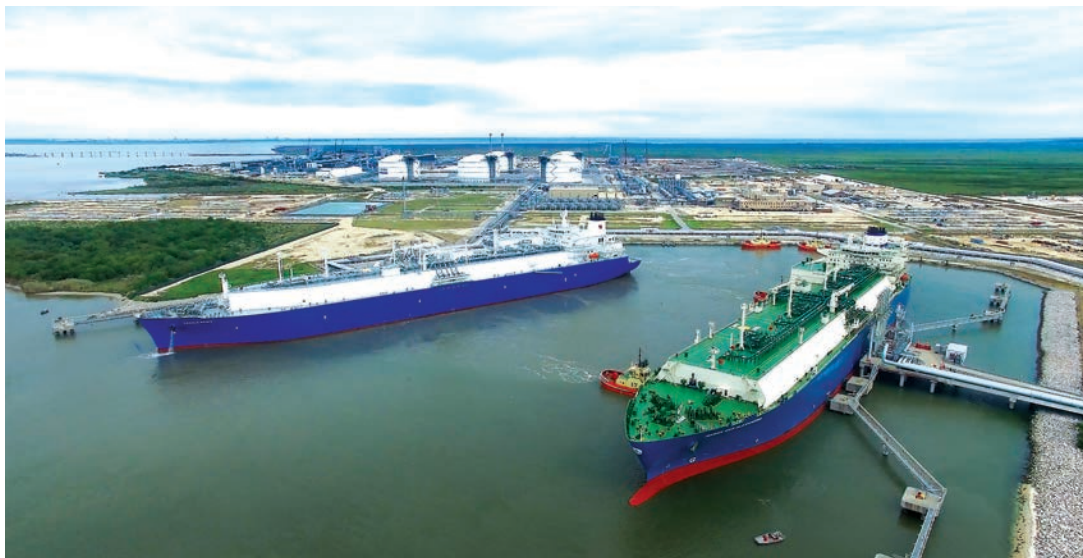
Two tankers take on liquefied natural gas at Cheniere Energy's ground-breaking LNG export terminal, built on 1,000 acres along the Texas-Louisiana border. Photo courtesy of Cheniere Energy
